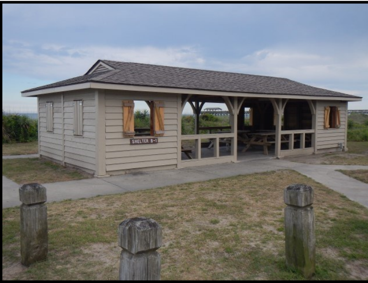
Shelter B1 Front View
